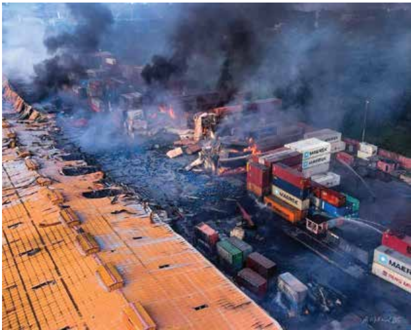
Picture of Chittagong Depot Fire Explosion
